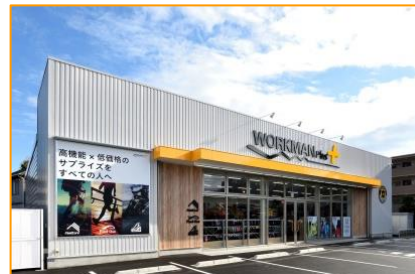
WORKMAN Plus at the roadside
